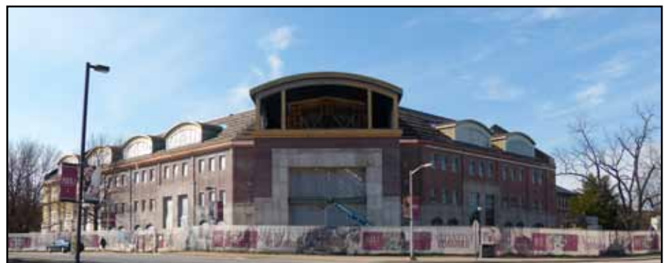
New Student Services Building under construction on SIU Carbondale campus.
