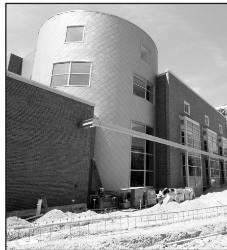
The new north face of Morris reflects the addition of about 50,000 square feet of space.
